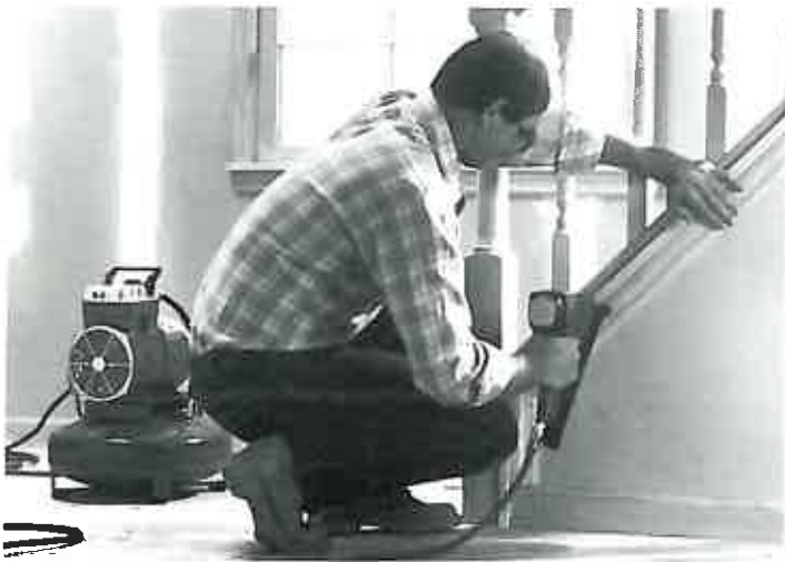
Small ½ H.P. compressor powers SFN1 to countersink or flush drive true brad-head nails.
