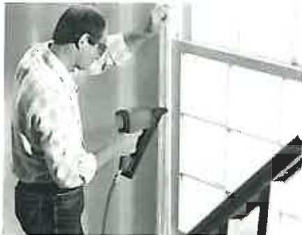
Window casings install rapidly with quality finish look.
